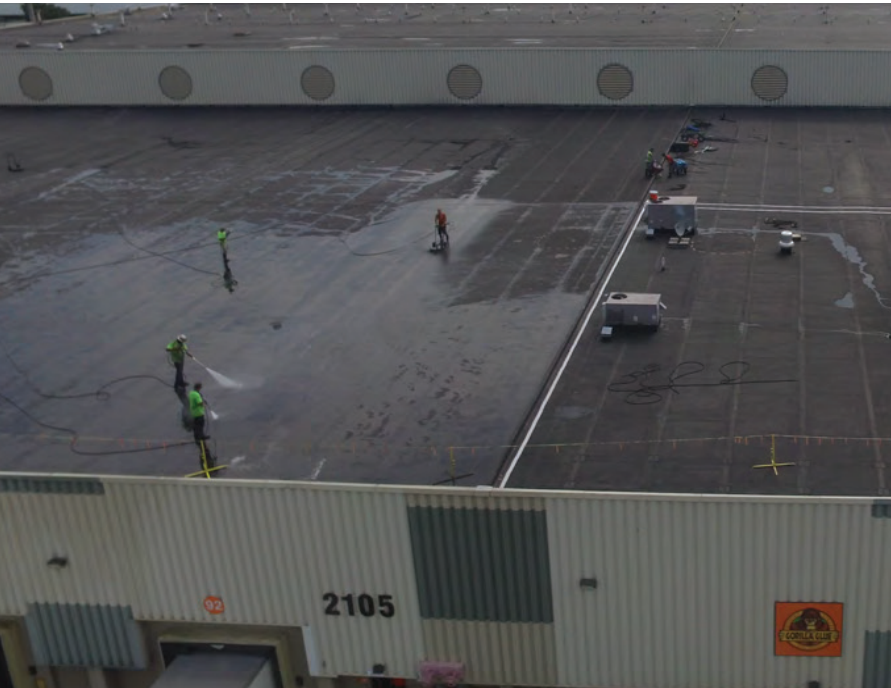
The entire roof had to be powerwashed to clean off a black substance present on many EPDM roofs.
