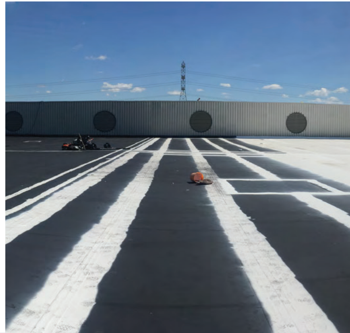
A halfway-coated black roof illustrates the benefits of a reflective roof, as you can see the difference in brightness on the wall.
